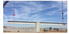
In all, 292 girders will be installed for the Salt River bridges. The girders, which serve as support beams, are manufactured locally and placed during overnight hours.
